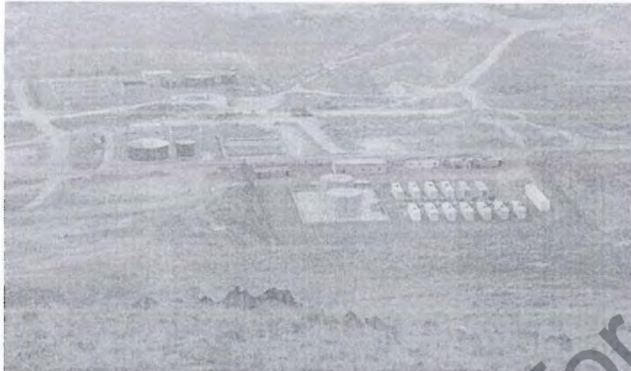
Existing Power Generation Plant
