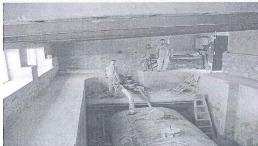
Buried Tanker Storage Tank
